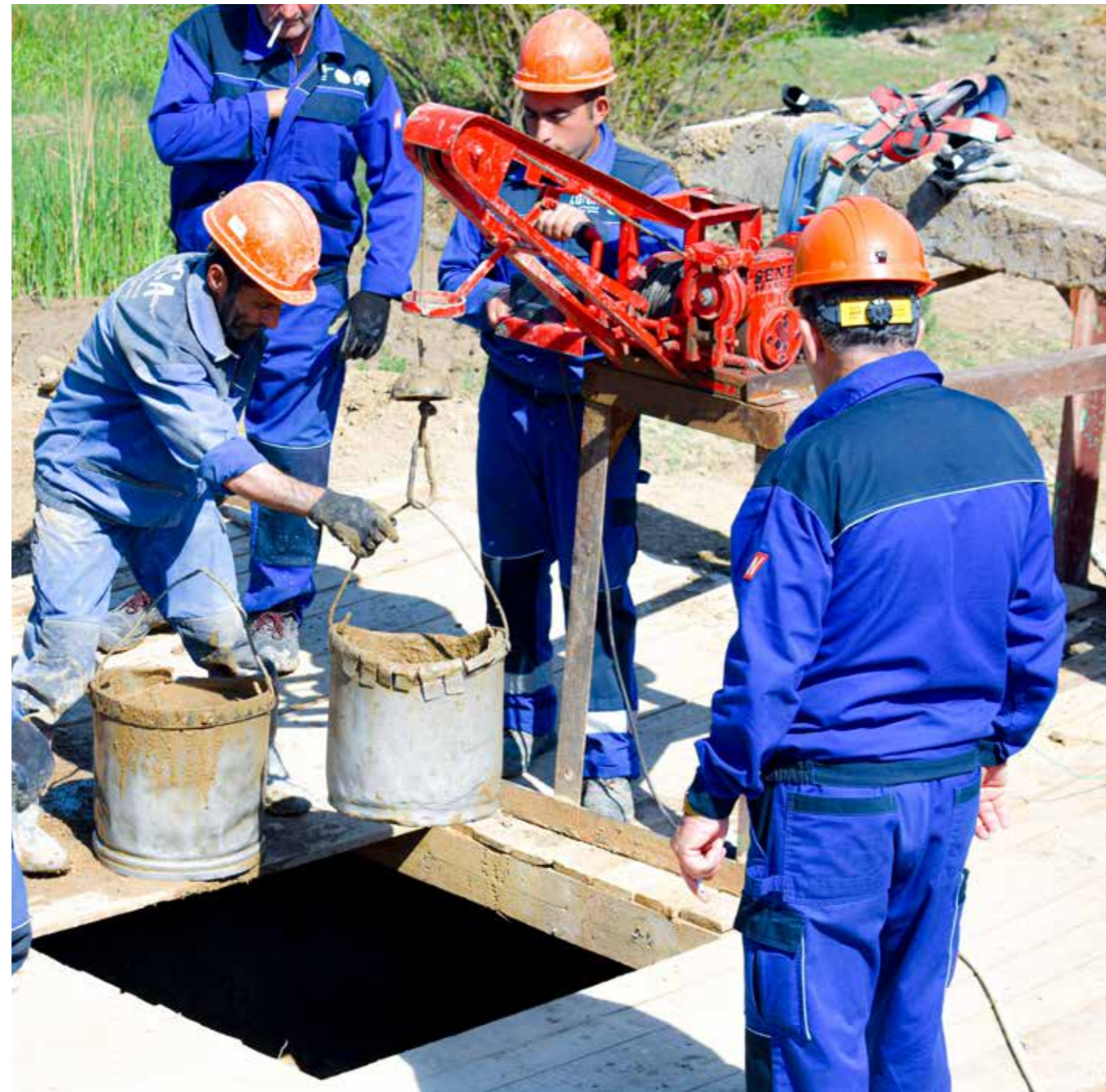
Rehabilitation works expands in ancient kahrizes- traditional, sustainable water supply systems. Photo credit: IOM/2022
